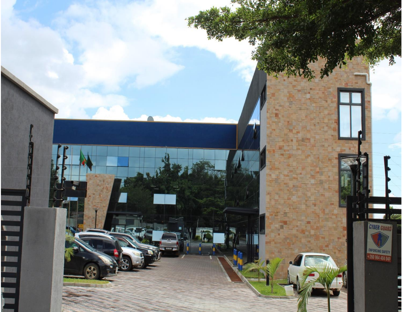
Newly built-fit-for-purpose HPCZ Head Office situated at Plot 6640 Mberere Road, Olympia Extension, Lusaka.
